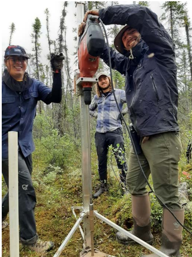
Members of the research team drilling in Whati to install temperature sensors for permafrost monitoring in 2022. (Credit: S. Wright)
